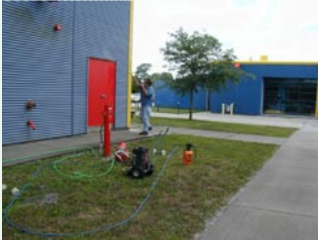
Figure 3. Periodic pressure washing of the building exterior and walkways is one way to minimize the amount of soil tracked into the building.
